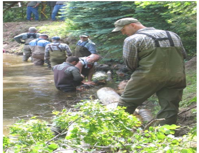
South Branch work site
