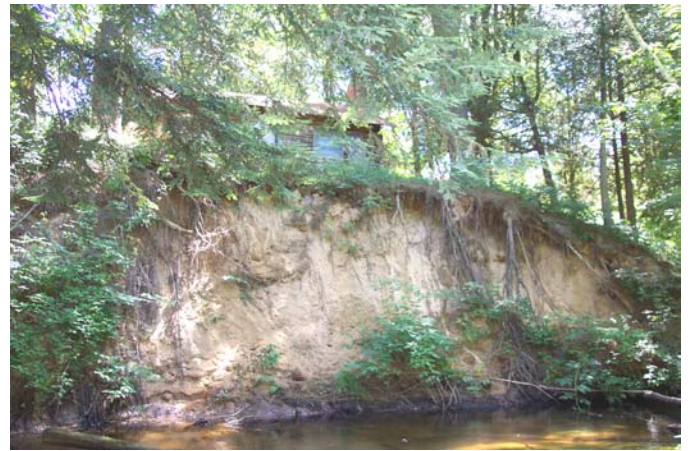
“ Before - Severe erosion and nearly vertical sandy banks are characteristic of the problem sites being addressed through the Headwaters project.”
